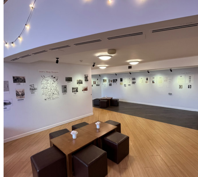
Ground Floor Entrance services includes radiator heating along with sidewall and linear diffusers for ventilation. Down lights and surface mounted light fittings.
