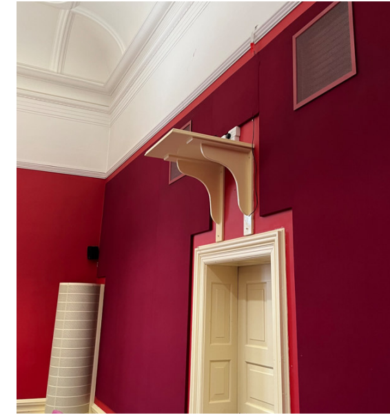
Council Chamber services are fed via air terminals providing pre-tempered air into the space via sidewall diffusers and dedicated ventilation pillars within corners of the room.
